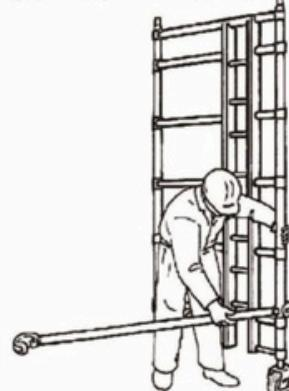
Fixed the cross bar on ladders horizontally, make ladders can stand automatically, the opening of lock at both ends of the cross bar must be outward.
